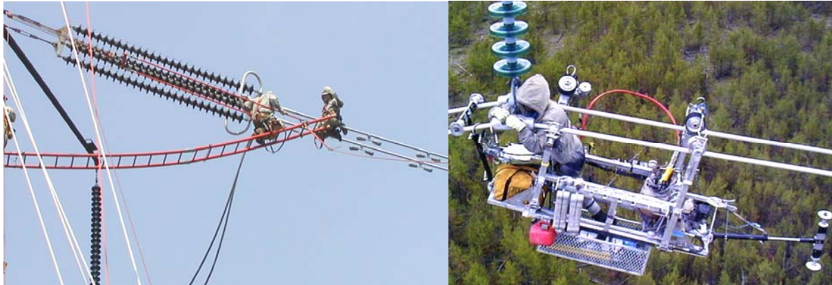
Figure 6 Service personnel working on energized lines.
