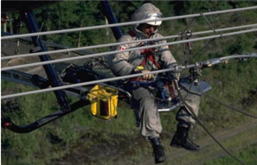
Figure 3 Replacement of failed splice (full-tension splicing of energized conductor).
