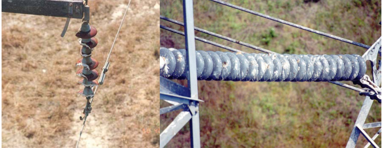
Figure 2 Insulators in need of replacement.
