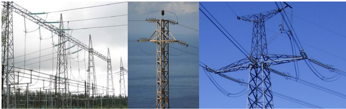
Figure 14 Difficult obstacles; a substation (left) and two tension clamps with creative cable loops.
