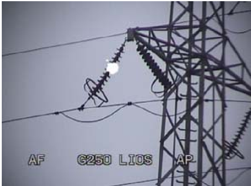
Figure 4 Corona on failing 150 kV porcelain insulator.
